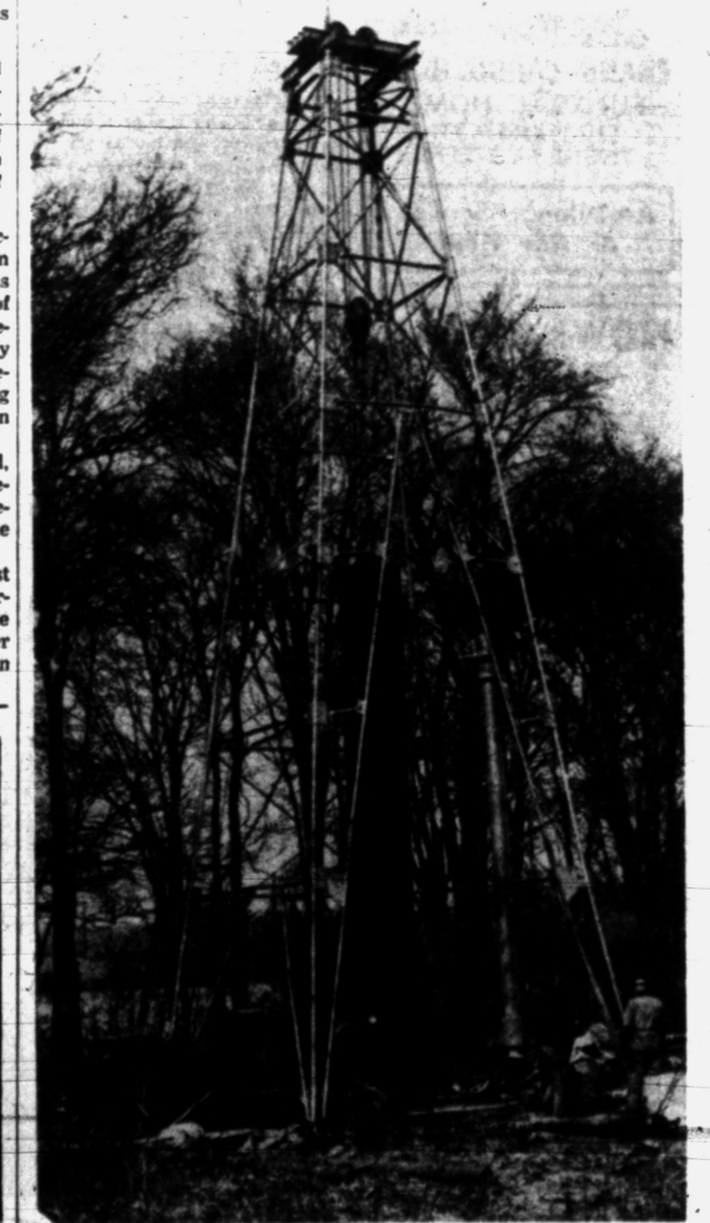
NEW CITY WATER WELL—A crew is shown drilling the first of three new water wells near Silver Lake. The wells are expected to up Pontiac's potential water supply about 25 per cent and produce an estimated 27,000,000 gallons a day. The wells will cost about $80,000. City officials hope the wells will be in operation before summer's peak demand.
