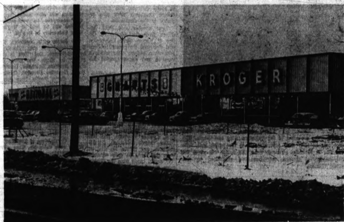
NEW SHOPPING AREA — Constructed in the last year, these three stores along with another row of stores west of them, make up the largest business district in White Lake Township.
