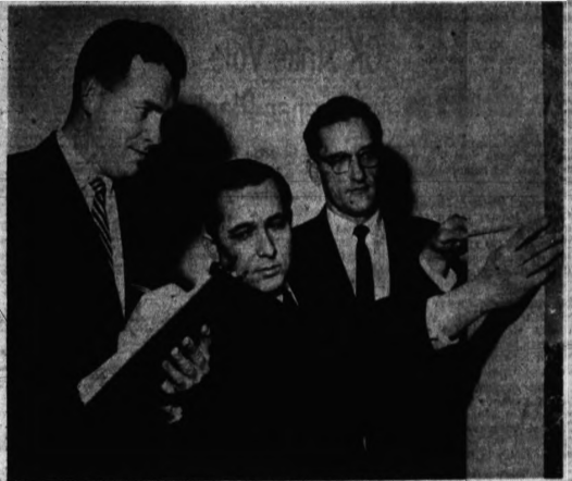
MASS MEASUREMENTS—Engineers began a physical survey of Pontiac buildings this week to determine the best potential locations for future community fallout shelters. William C. Bailey records the data as Theodore E. Kuhn measures the thickness of a wall at Pontiac General Hospital. Wall mass is a vital factor in the survey. Both men represent Giffels & Rossetti, Inc., Architects-Engineers, of Detroit, under federal contract to make the shelter survey in this area. Both have Department of Defense identification cards. Watching the procedure is Donald H. Carros, assistant hospital administrator.
