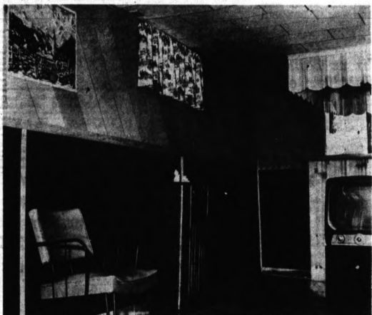
UNUSUAL WALLS — A brown leather-like material is used on the lower part of the walls with diagonal Celotex above. The latter has a rosy cast to it. Just a bit of the pine bar can be
