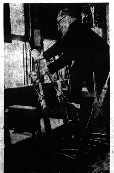
TAKES STRENGTH — That's what Earl Iles of Oxford thinks, as he pulls the big switches in the old tower near his station. Iles has taken over the responsibilities of the Drayton and Clarkston depots since they were closed for lack of customers. Oxford's is one of the busiest freight depots in Michigan.
