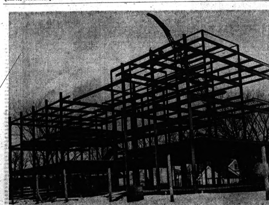
PONTIAC MEDICAL BUILDING — The skeletal structure of a new 25-story building created by and for doctors is now completed just across S. Johnson Street from Pontiac General Hospital. The 23,600 square feet of
