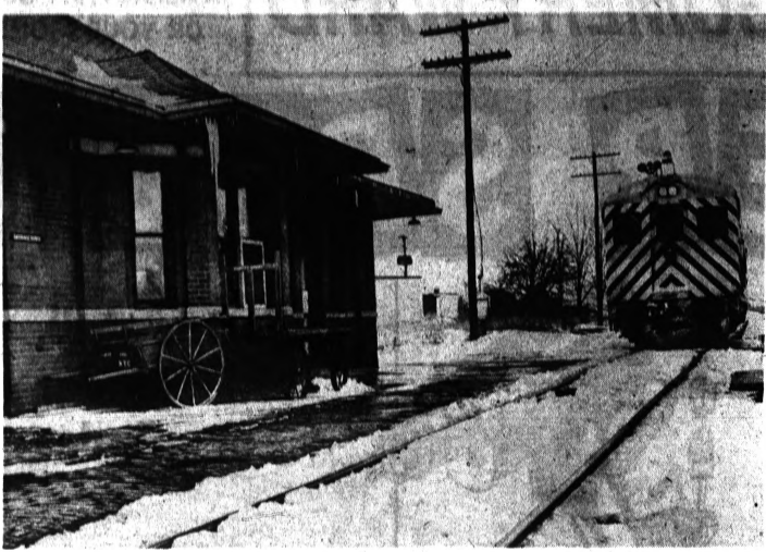
HEADING IN — This bug-like New York Central train is shown crossing the Grand Trunk railroad tracks in the heart of Oxford. Oxford's largest out-going freight load is sand and gravel. However, the one-car, "Doodlebug" above transports passengers.
