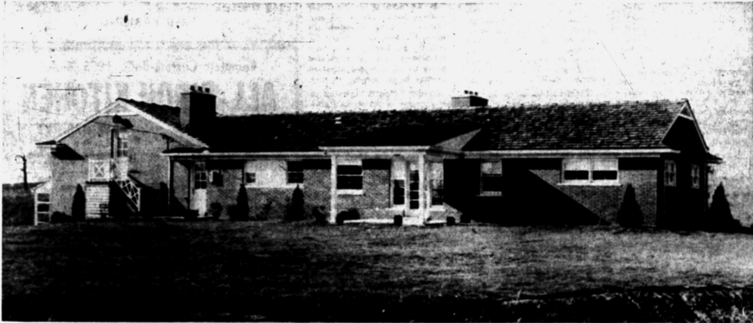
BACK VIEW OF RED BRICK —Built into a high hill in Canterbury Hills, the backview of the above house shows the two fireplace chimneys and three back entranceways. The one at the left leads to
