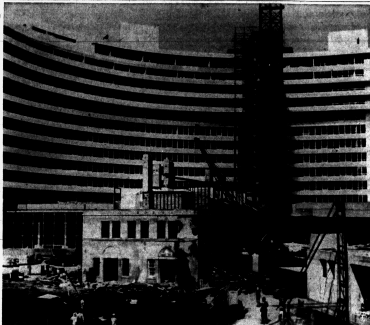
OLD FIRESTONE MANSION RAZED —A wrecker's crane works on demolishing the famous Firestone Mansion in Miami Beach, Fla., to make room for completion of the $14,000,000 Fontainebleau Hotel (in background). The formal Gardens of Versailles are to be reproduced in area where mansion now stands. The new hotel, scheduled for a December opening, will have 565 rooms.
