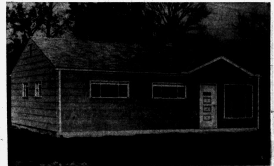
PASTEL ONE-STORY —Three bedroom one-story models with tiled bath, oil heat and constructed on large lots are being offered by Wright and Vallet of Pontiac. Located off White Lake Rd., the development is known as Jack's
