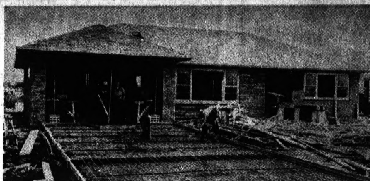
BEST TIME — While the house is being built is the best time to install a hydronic snow-melting system. Pipe coils are laid down first, becoming embedded in the concrete or
