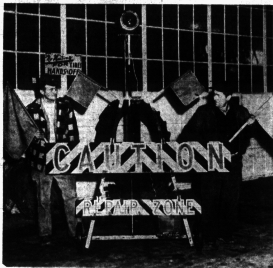
ROAD COMMISSION WARNING —Workmen Louis McDonald of Davisburg, left, and Bert Dickens of Lake Orion put the flags in a new caution apparatus developed by Oakland County Road Commission to safeguard its road crews working in high-speed traffic. The sign, 6 feet wide, features a police-type flasher signal, battery powered, on a collapsible pole 10 feet high.
