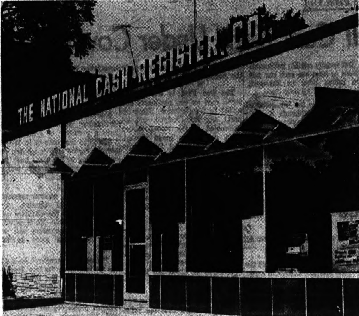
SPORTING NEW LOOK —Most noticeable of the extensive renovations to the National Cash Register Co. quarters, 562-64 W. Huron St., is the newly remodeled front. Building improvements include an enlarged service department and more demonstrating rooms.
