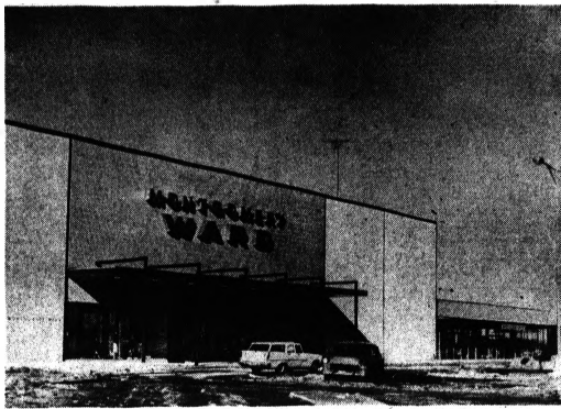
FRONT VIEW OF WARD'S—Viewed from the front facing North Telegraph Road. Montgomery Ward's new store in the Pontiac Mall Shopping Center displays a wide-awning-like porch top over its front entrance. The cream-colored brick construction, accented by turquoise lettering en-
