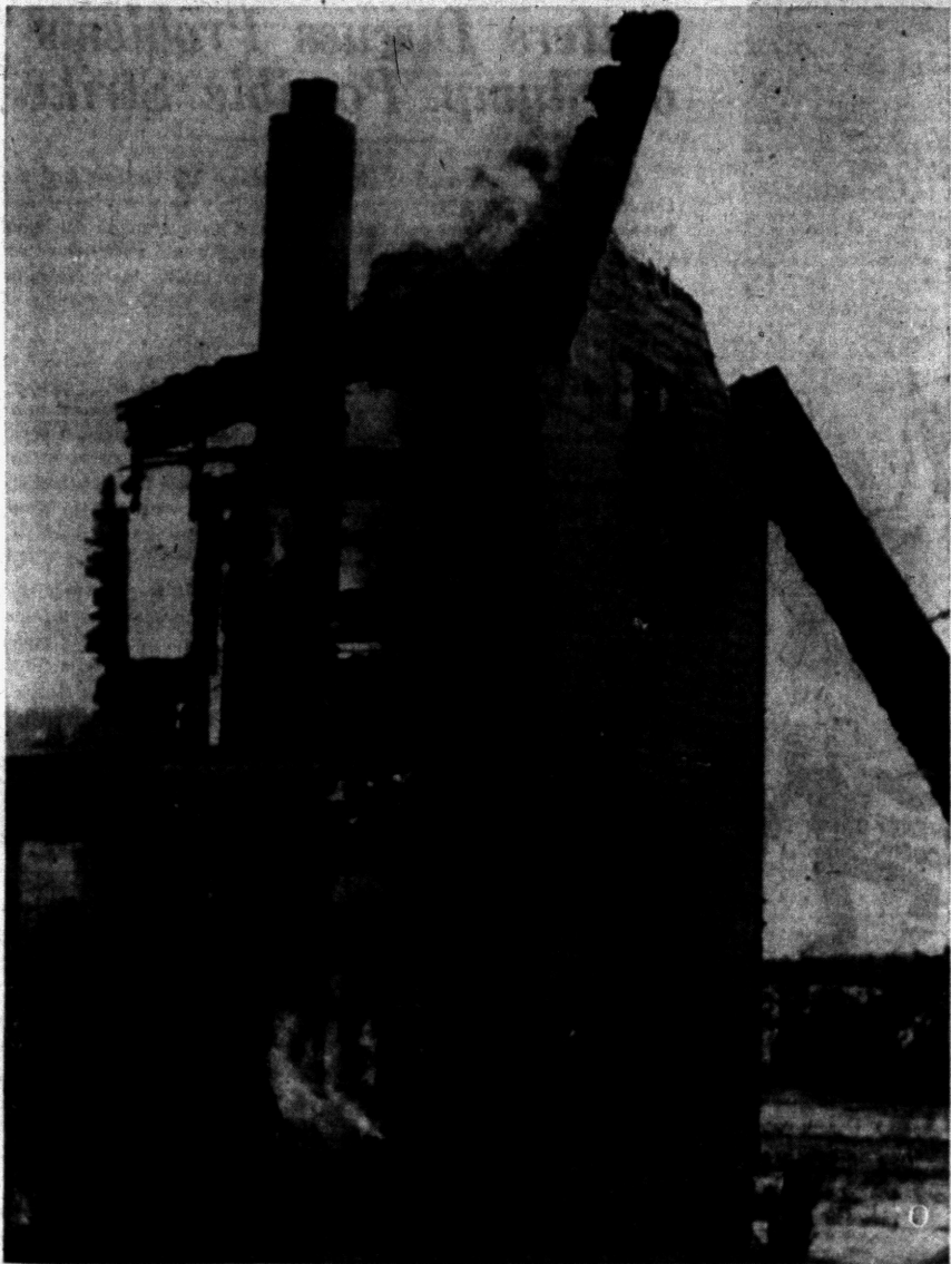
ORTONVILLE HOME DESTROYED — Four fire departments battled this blaze which destroyed the Virgil Hickey home, 700 State Park Rd., Ortonville, shortly after noon yesterday. Much of the family's furniture was saved, but nothing was left of the house except the chimney. Brandon Township Fire Marshal William Buckingham said the fire apparently was caused by faulty wiring. Other departments fighting the blaze were from Atlas and Independence townships and Oxford Village. Firemen said, however, that the house was a mass of flames when they arrived — too late to be able to stop it.
