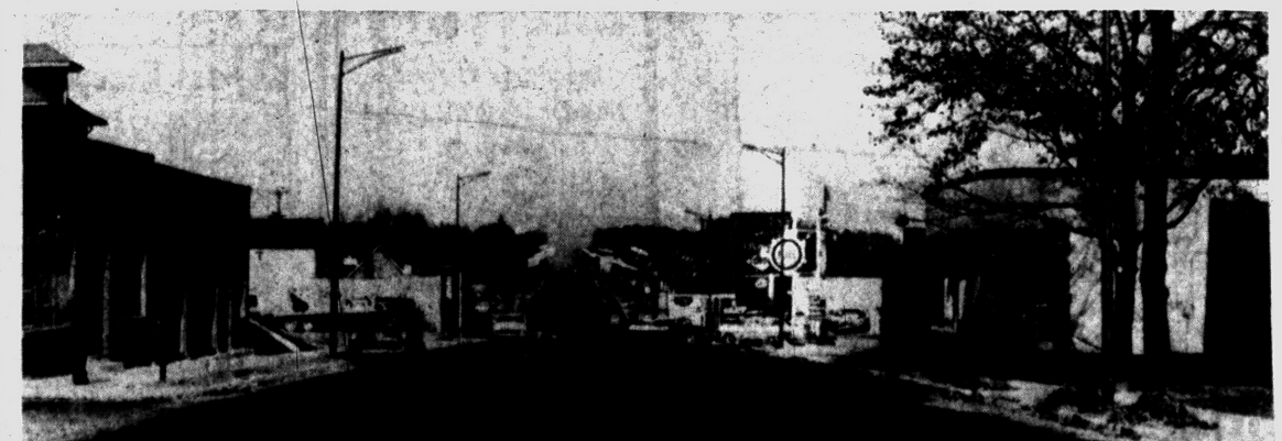
WIDENED PERRY STREET — This is how the newly widened Perry street looks to a motorist driving out from downtown, at the
