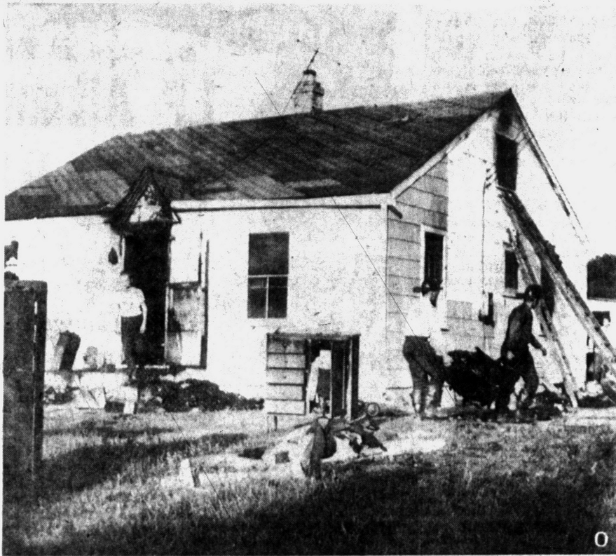
GUTTED BY FIRE — The home of Mr. and Mrs. John E. Schirmer, located at 4857 N. Rochester Rd., Leonard, was gutted by fire at 4:30 this morning while the whole family, except Mrs. Schirmer's brother, Robert Trufant, were on vacation. The blaze leaves the Schirmers, who have six young children, homeless. Mrs. Schirmer's mother lives with the family, but she also was away today.
