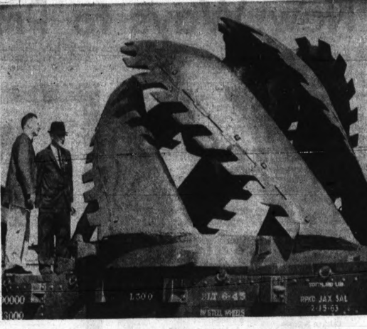
FAIR BITE — This 55,000-pound cutter head for a dredge left Jacksonville, Fla., recently for Long Beach, Calif., where it will dredge up land for the site of the 1967 World's Fair. Two more will soon be sent along.
