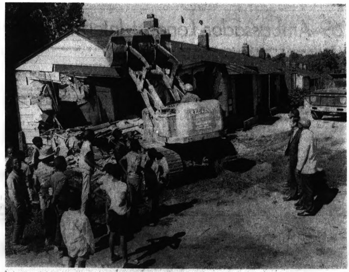
GOING DOWN — Demolition of eight units of the Crystal Beach housing project attracts a number of area youngsters yesterday. Also on hand were District 1 City Commissioner T. Warren Fowler Sr. (at right, white coat), building inspector Robert Gerds, and James Egglestone, a resident of the project.
