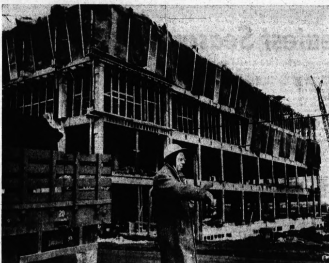
SPROUTING NEW BUILDING — Despite the wintry weather signs lately, work crews on the county's new $3,000,000 courthouse in the Telegraph road Service Center move ahead. On the other hand, the architects have had to plow through some complaints from department heads. Here watching workmen move ahead on the fourth floor frame of the six-story building is George Kimber, county project engineer.
