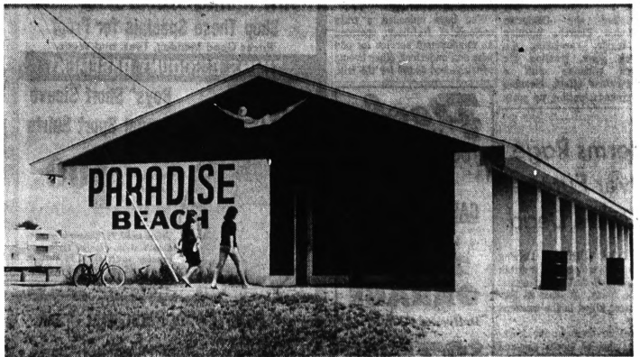
Beach House Contains Refreshment Stand, Offices
