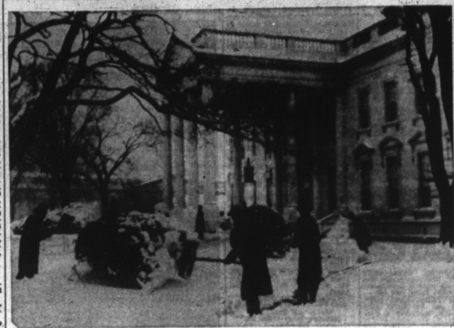
WHITE HOUSE REALLY WHITE —Workmen at the White House shovel paths clear of now at the height of a storm Friday which blanketed the Washington area with more than eight inches of snow. It was the district of Columbia's worst storm in recent years.
