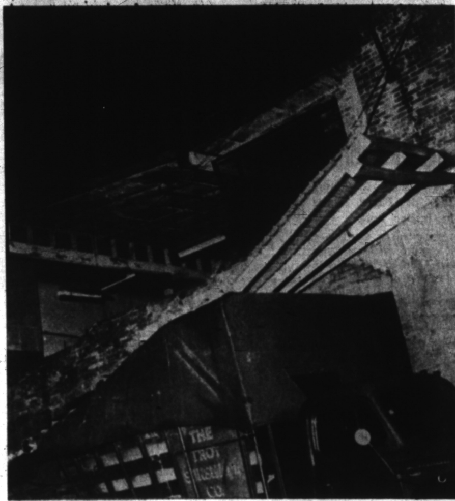
TORNADO DAMAGE — This picture from Troy, Ohio, shows a caved-in section of a second floor wall of the Troy Sunshade Co., which was in the path of a
