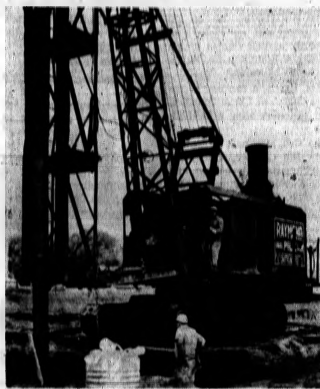
OBJECT OF FIE — Lake Oakland Heights residents have secured a temporary restraining order against use of this pile driving machine at the nearby water tower construction site to the extent that it causes damage to their houses. While attorneys for the residents and for Waterford Township and Oakland County are in court today regarding a show cause hearing on the injunction, the machine is still in operation.
