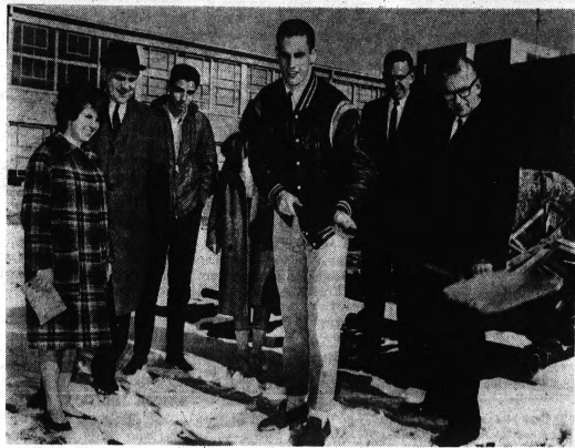
SCHOOL PROJECT STARTS —Dale Jones, student council president at Waterford Township High School, handled the shovel yesterday during ground-breaking ceremonies for the school's $500,000 addition. Looking on (from left) are Karl Haaset, council vice president; Dr. Don O. Tatroe, superintendent
