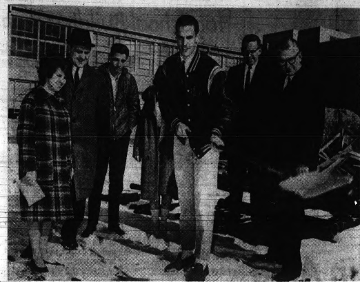
SCHOOL PROJECT STARTS —Dale Jones, student council president at Waterford Township High School, handled the shovel week-day during ground-breaking ceremonies for the school's $500,000 addition. Looking on (from left) are Kari Haaset, council vice president; Dr. Don O. Tatroe, superintendent of schools; Mike Skelton, council treasurer; Paul O'Neill, school principal; and Barrett Vorce, assistant superintendent for general administration. Partially hidden behind Jones is Carol Parker, council corresponding secretary. (See story, page 2.)
