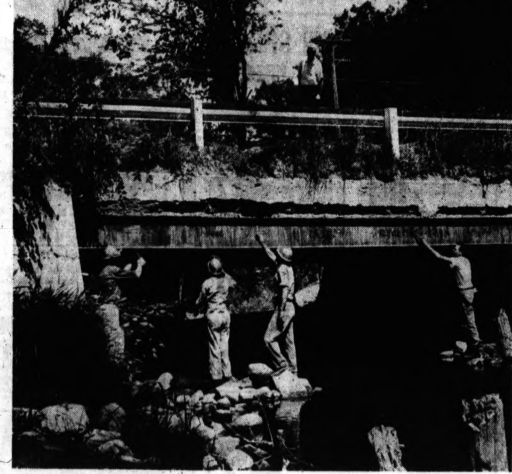
BRIDGE FACE-LIFTING — The timing is just right for the Oakland County Road Commission maintenance crew to clean and paint a bridge over Paint Creek. It ties in with "Operation Clean-Up" of the stream bed which will get under way Aug. 15. Here Oakland Township team captain C. H. Williams watches from the bridge as rust-scraping work begins. The bridge is over the creek on Orion Road at Snell Road.
