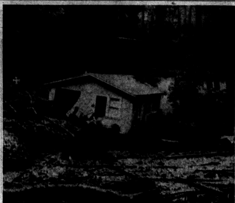
MUD MOVES HOUSE —A house in the Oakland hills of California dips at a crazy angle after heavy rains loosened tons of dirt and trees. A woman and her son were in the house when the mud hit, but escaped uninjured. More than four inches of rain fell in the area over the weekend.
