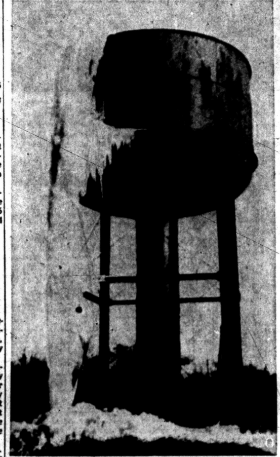
ANYONE WANT AN ICE? — Biggest icicle in Bay County forms on the water tank at the Michigan Central Railroad North Euclid yards in Bay City. A railroad spokesman blamed the frozen overflow on a minor leak in the tank's wall, indicating repairs will be needed as soon as the tank can be drained.
