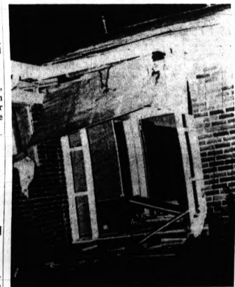
DAMAGED HOME — A pre-dawn blast today ripped off the front door and severely damaged the home of Fred Alexander, a Negro leader and member of the Charlotte (N.C.) City Council. The homes of three other Negro leaders, including Alexander's brother, were also damaged by explosions.
