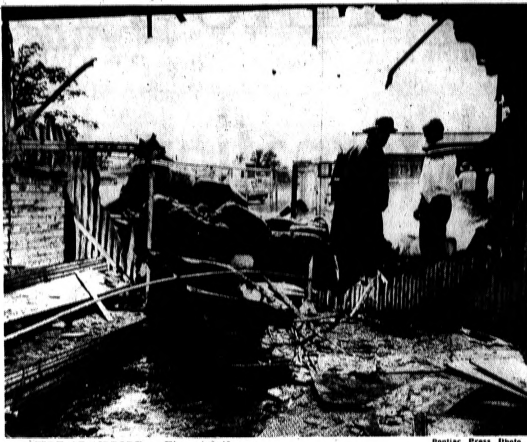
FIRE AT AIRPORT — Fire at 2:40 p.m. yesterday caused an estimated $2,000 damage to the Carl Strand Wood Products Co. building, adjoining Barber's Flying Service at the Pontiac Municipal Airport. A trash fire in an open container at the west side of the building ignited several fiber glass tubs stored nearby, according to Waterford Township Fire Marshal Russell See.
