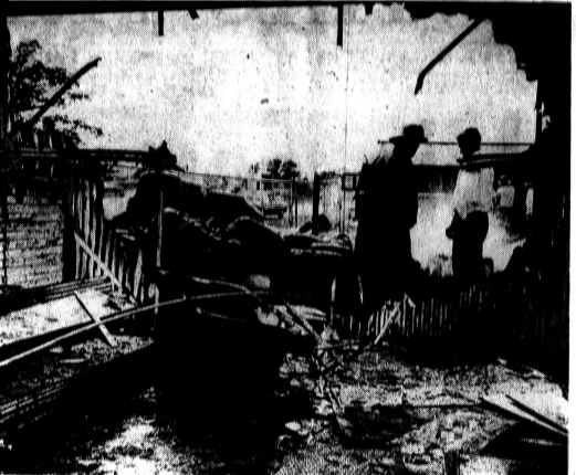
FIRE AT AIRPORT — Fire at 2:40 p.m. yesterday caused an estimated $2,000 damage to the Carl Strand Wood Products Co. building, adjoining Barber's Flying Service at the Pontiac Municipal Airport. A trash fire in an open container at the west side of the building ignited several floor glass bins stored nearby, according to Waterford Township Fire Marshal Russell See.
