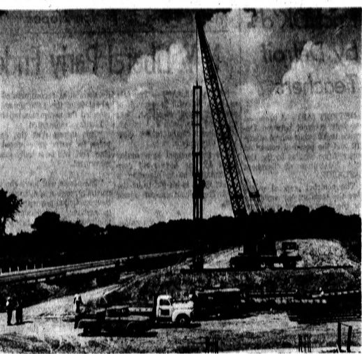
HIGHWAY CONSTRUCTION — Work began last month on the third section of the 10.5-mile-long, $11.5 million M59 Freeway along Adams Road just north of Auburn. Completion date for the third section of the freeway, which will connect Pontiac and Utica, is November. The second section, from the Grand Trunk Railroad to I-75 is nearly complete. Contracts will be let in 1966 for work from Wide Track Drive to the railroad.
