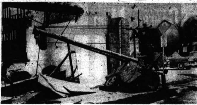
THIS IS VERY UPSETTING — Looks like a draw in this contest between a 1½-ton "T" beam and a Flint wrecking company truck. The truck managed to lift the beam off the walls of a Flint building Thursday but the weight of the beam tipped the truck. All
