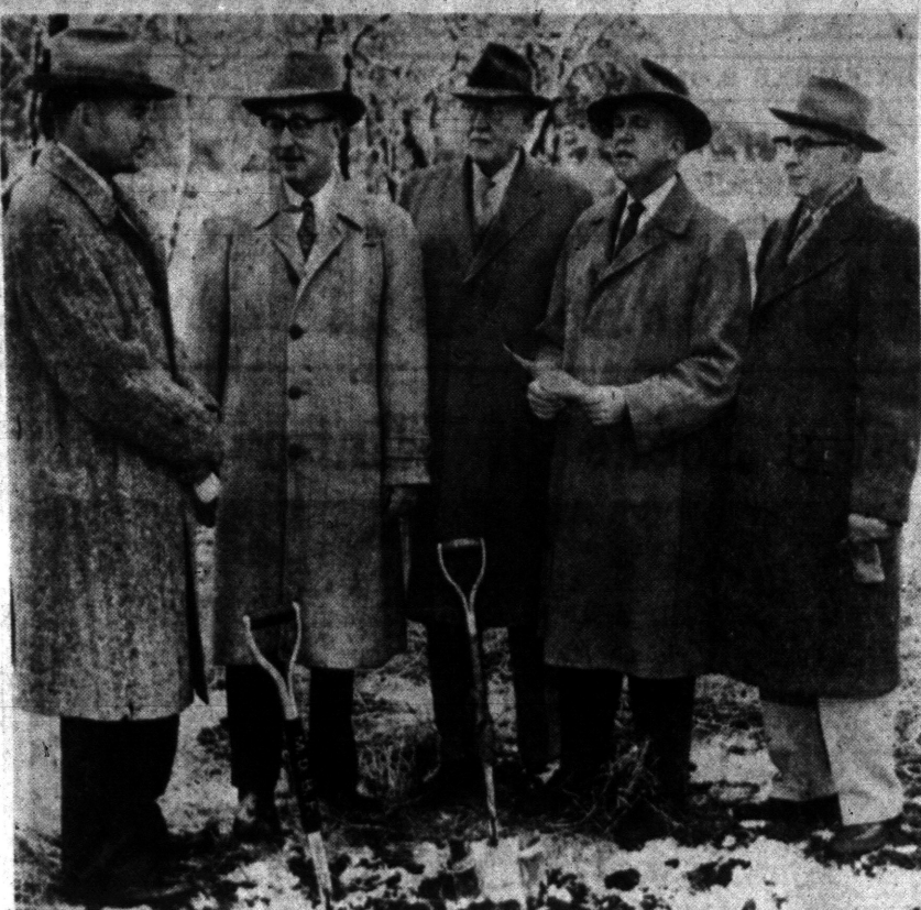
BREAK GROUND FOR NEW YMCA — Birmingham's new YMCA branch will soon be a reality. Ground breaking ceremonies were held yesterday afternoon and construction work on the $144,000 building at Lincoln and Edgewood avenues is expected to begin immediately. Participating in the ceremony Sunday are, left to right: Everett Allen of the Building Committee; Col. Leslie Fletcher, chairman of the Board of Management; Dr. John K. Ormond of the Board of Management; Edwin F. Kirbitt, executive secretary, Board of Management; Joseph R. Dingley of the Board of Management; and W. C. Gordon, co-chairman of the Building Committee.
