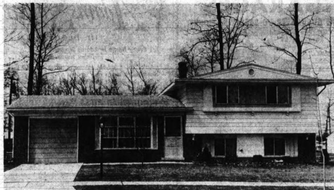
YARD LIGHT — A black, wrought-iron gas light in Mrs. Marjorie Hellner's frontyard on Buffalo Drive, Commerce Township, gives a hint of the home's traditional interior. The
