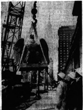
EVICTED EAGLE — After 53 years of gazing down on the traffic from its "nest" on New York's Pennsylvania Station, this 5,700-pound granite eagle is swung out of its nest and lowered to the street by a huge crane. The eagle—one of a "family" of 13—is making way for a new sports arena.
