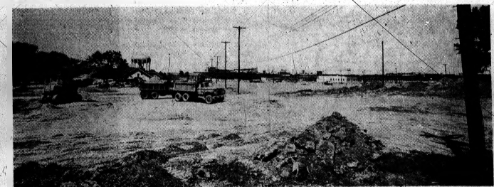
Site Of New 25-Acre Parking Lot Under Construction At Pontiac Motor Division
