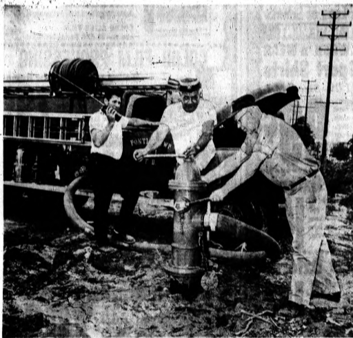
TO THE RESCUE — Pontiac Township firemen from Station No. 1 in Auburn Heights were asked to perform unusual duty the past couple of days. They manuevered a fire hydrant on South Boulevard to provide extra water to a main in Bloomfield Orchards Subdivision.
