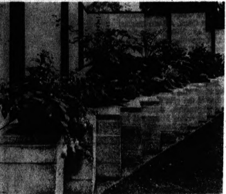
NEW STYLE — Raised planter set in a saw-toothed pattern puts planting bed at a height that makes it easy to tend. Rustic faced concrete block merges quietly with the surroundings.
