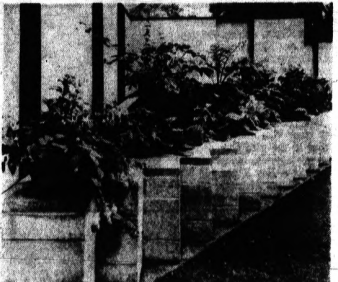
NEW STYLE — Raised planter set in a saw-tooth pattern puts planting bed at a height that makes it easy to tend. Rustic faced concrete block merges quietly with the surroundings.
