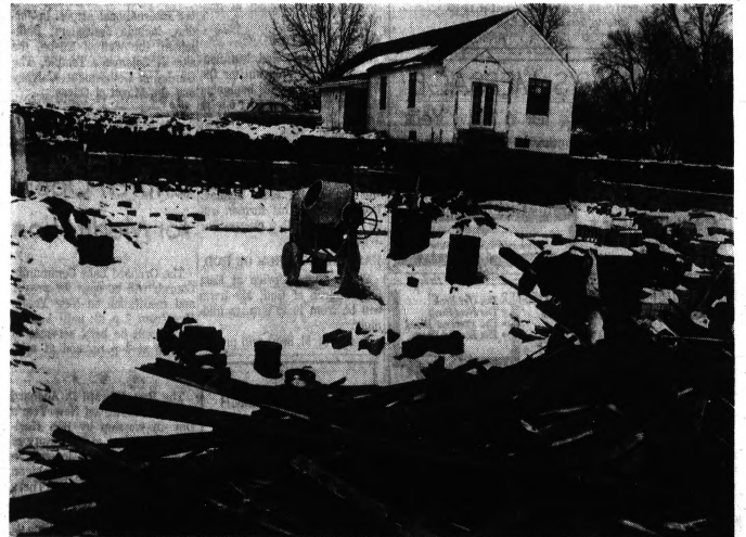
BEGIN BASEMENT —Walls of the basement of the new Elizabeth Lake Church of Christ are going up at 183 S. Winding Drive, Waterford Township. The present building in the background will be used as an educational unit when
