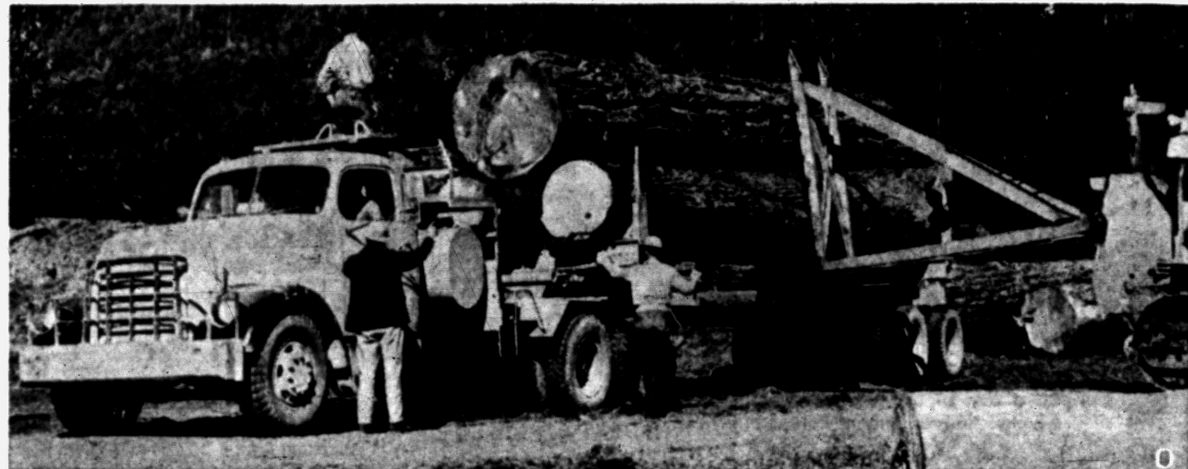
TRUCK AND COACH DISPLAY —A logging vehicle similar to this diesel-powered D970 GMC tractor-trailer combination will be displayed by GMC Truck & Coach Division at the General Motors Powerama in
