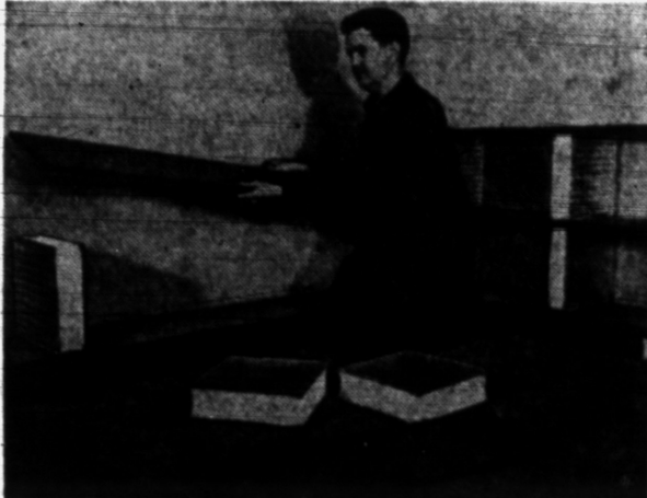
STEP NUMBER TWO —The finished shelves add a smart modern note to the room. You need have no worry about the strength of the shelves, because the glass blocks used are made for structural use. Blocks laid on their sides raise the bottom shelf from the floor. The shelves are easily dismantled and moved.
