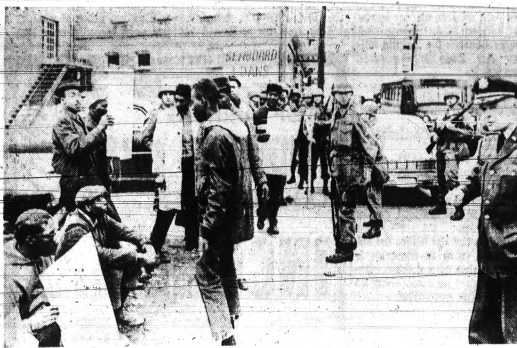
HALT DEMONSTRATION — Brig. Gen. George G. Gelston (right) tells Negro demonstrators yesterday they have broken Maryland
