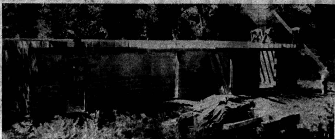
ANIMAL SHELTER PROGRESSES — Roof was being started on the Michigan Animal Rescue League shelter at Featherstone Rd. and East Blvd. when this picture was taken. The building is expected to be ready for use before end of the summer. It will have five rooms and is 22x60 feet in size. Much of the material has been donated and labor for building the room was donated through efforts of Grady Pinner, representing the Carpenters' Union; Gordon Coughlin, contractor, and Robert Chapin, Stephen Rebb and Philip Mutersbaugh.
