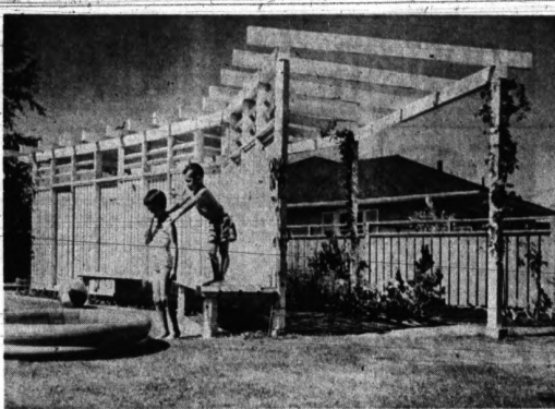
WINSOME ARBOR —Delightful yard accessory is this angled arbor which screens a cutting garden. Built of white painted Douglas fir, the arbor is simple to construct. Four-by-fours are the main supports, and posts are set on concrete bases to keep them free of the ground.
