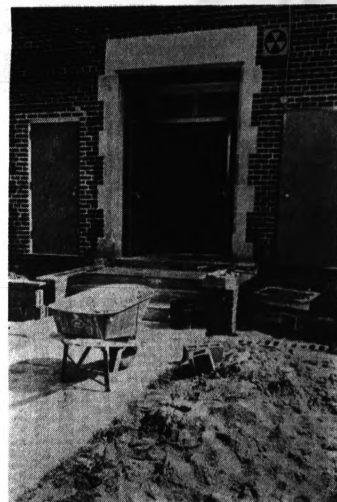
FIRE DOORS —These three doors were put in place on the orders of the state fire marshal. The former Youth Home did not have enough exits to meet the fire regulations for a large number of students in individual rooms. Thus, these doors had to be hacked out of the brick.
