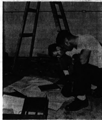
CHECK PRINTS —Ed Barnett (left), superintendent for Moote Electrical Co., and Laine Heitherington, foreman, check blueprints for remodeling of a room slated to be a recording laboratory for the new community college campus.
