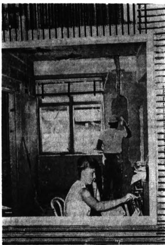
BUSINESS AS USUAL —Switchboard operator Mrs. Brian Marchant of 5901 Dixie Highway, Independence Township, can clearly take claim to the title as the first person to occupy projected offices in the old hospital building at the new Highland Lakes campus of Oakland Community College. She operates her switchboard amid remodeling work being done there.
