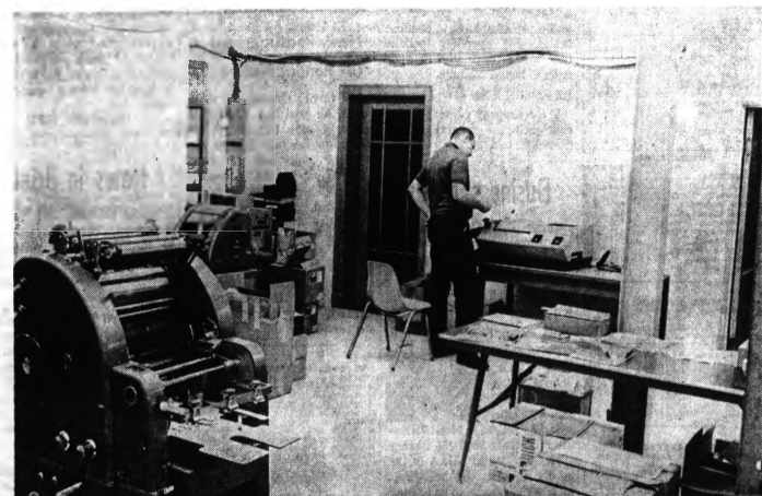
DUPLICATING AREA —Printer James Richardson operates some of the initial equipment moved into the basement of the administration building at Highland Lakes campus.
