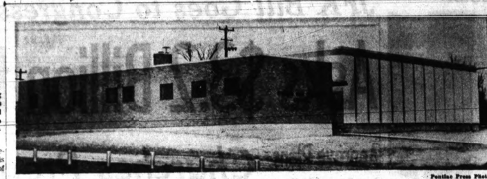
Modern New Plant—Michigan Bell Telephone Co. will put its new $14,100,000 plant on Cass-Elizabeth Lake Road in Waterford Township into operation early Sunday morning. At that time 6,700 customers west of Pontiac will be switched over to the new building to relieve the downtown office and allow for future expansion. Customers involved in the switchover also are being assigned all numerical telephone numbers, eliminating the FE suffix. (See story on Page 1.)
