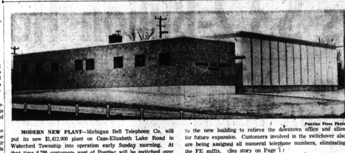
MODERN NEW PLANT—Michigan Bell Telephone Co. will put its new $1,412,000 plant on Cass-Elizabeth Lake Road in Waterford Township into operation early Sunday morning. At that time 6,700 customers west of Pontiac will be switched over to the new building to relieve the downtown office and allow for future expansion. Customers involved in the switchover also will be assigned all numerical telephone numbers, eliminating the FE suffix. (See story on Page 1.)
