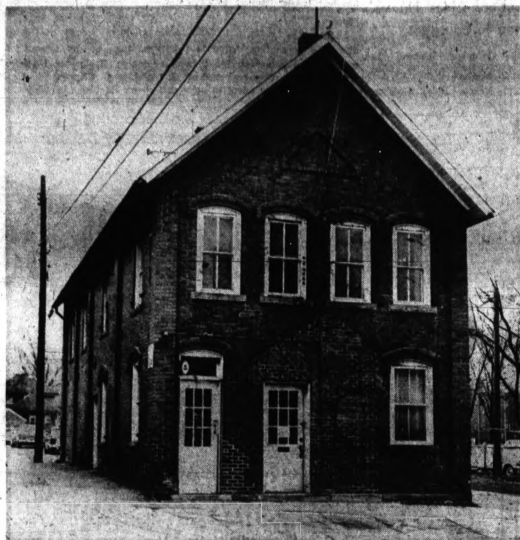
TO BE RAZED—The old municipal building which has served the village of Rochester for 67 years has been condemned and ordered torn down. Demolition work on the two-story brick structure which was built back in 1894 for $1,400 is slated to begin early next week under the direction of Thomas J. Turkette, Rochester's chief building inspector. The village offices, council chambers and police department now are housed in a new $100,000 municipal building in Stone Park which opened two weeks ago.
