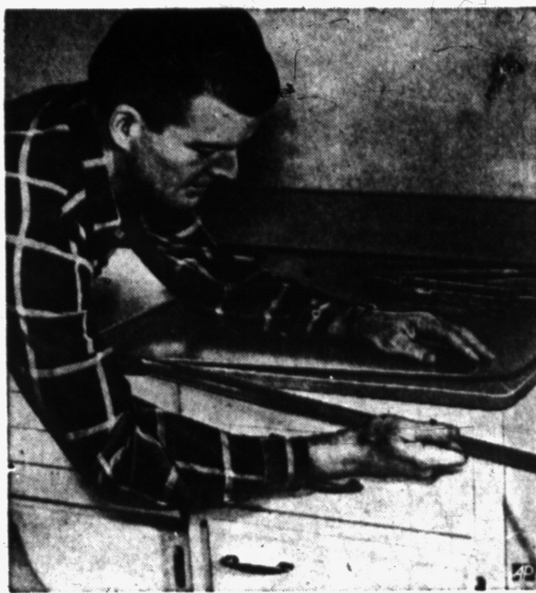
CUPBOARD TOPS —New thin plastic covering for countertops is curved to make it lie flat under tension from metal trim.
