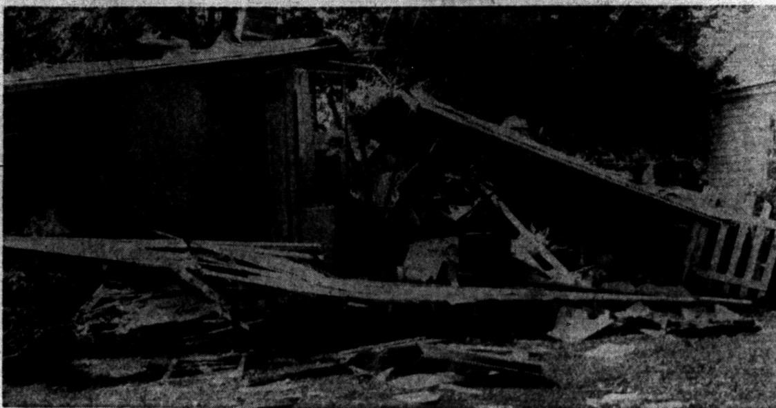
SMASHED KEEGO HOME — Mrs. Gloria Bray, of 2918 Virginia Ct., Keego Harbor, was pulled from the wreckage of her home this morning, after a gas explosion demolished it. She was
