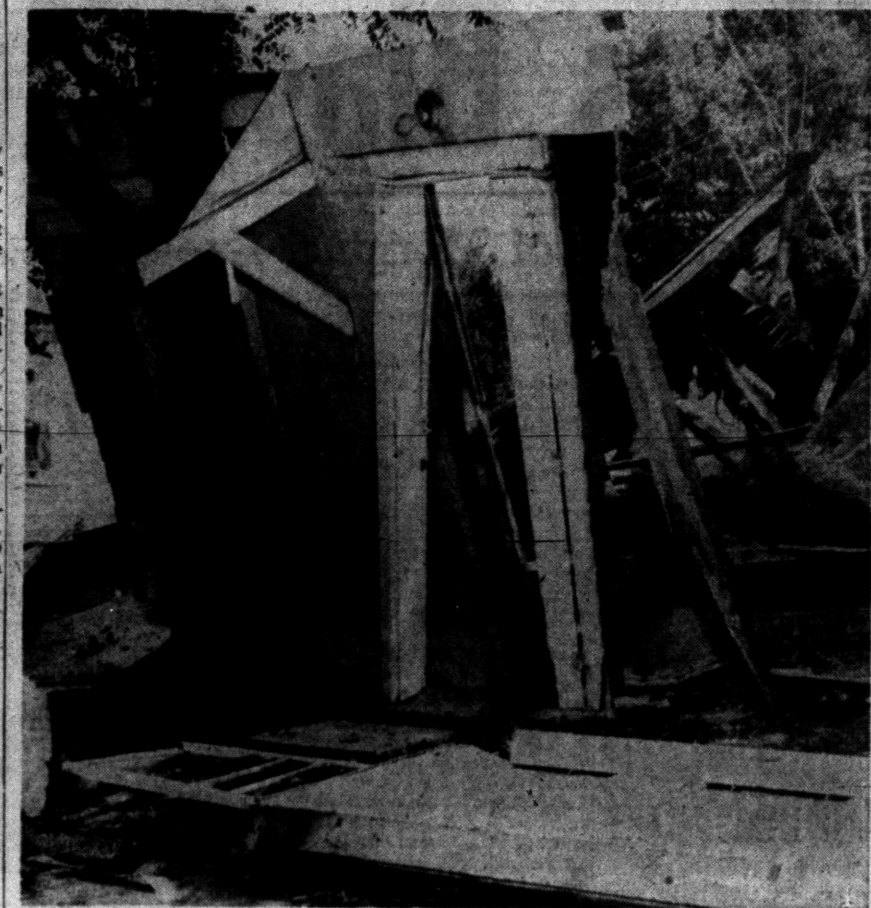
LEANING FRONT WALL— This front section of the 2918 Virginia Ct. Keego Harbor residence of the Brays was blown up against a front yard tree by the force of the blast which smashed their home this morning. The blast was heard more than two miles away.
