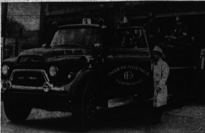
WELCOME ADDITION — Independence Township Fire Department's new fire engine passes a final inspection by firemen and members of the Township Board with flying colors. Fire Chief Donald Beech prepared to put the $20,000 vehicle through its paces with firefighters Frank Green and William Wilson aboard. Shown
