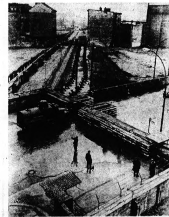
NARROW BORDER GAPS —This overhead view shows how the Communists have narrowed gaps in the wall at Berlin's Heinrich Heine Strasse checkpoint between east and west sectors of the divided city. A water truck is at the entrance into West Berlin. At right is the cramped entrance for people before which are standing East German policemen. In the background are steel tank traps in the East German sector.
