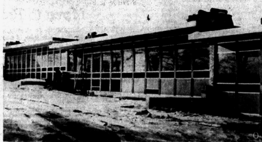
SCHOOL CONSTRUCTION ON SCHEDULE—Workmen install windows and panels in new Romeo High School as construction moves toward completion.
