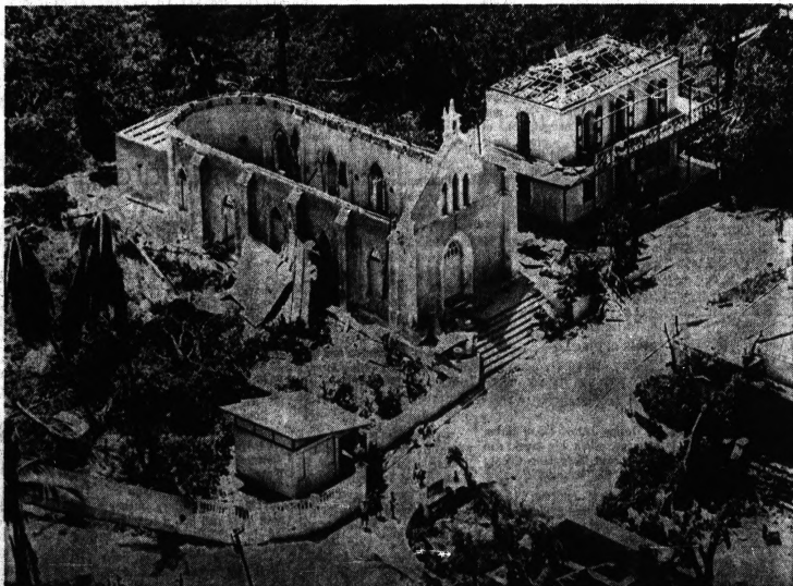
ROOFLESS CHURCH—The force of Hurricane Inez ripped the roofs from this church and house next door in Jacmel, Haiti, last week and it is feared that nation hundreds of persons are dead
