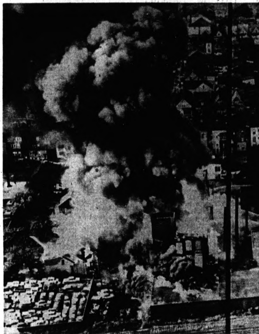
PLANT WRECKED — Flames and smoke billow from burning textile dyeing plant yesterday in Paterson, N.J. Gas explosions touched off the spectacular blaze. Twenty-eight persons were injured and one is missing.
