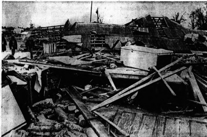
DIXIE TORNADO—One of the random tornadoes which swept across middle Georgia last night shattered this frame house north of McDonough. The area in Henry County was
