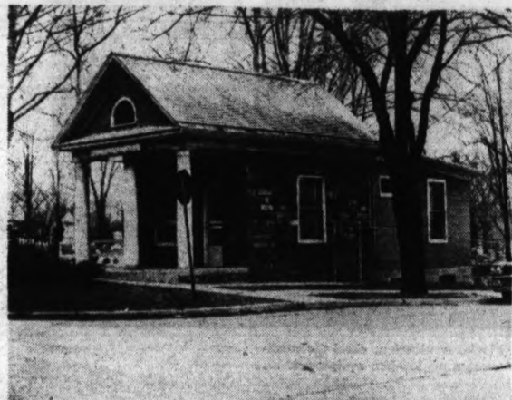
The new addition to the Oak Hill Cemetery building provides much-needed reception area and office space.
