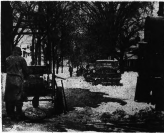
DPW crew rods a sewer . . . over 33,000 lineal feet were rodded and dragged in 1959.
