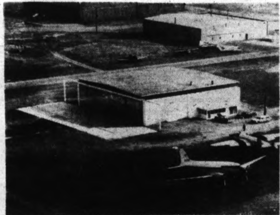
New $80,000 Hangar and offices of Festa, Inc., located in the corporation hangar area of Pontiac Airport.
