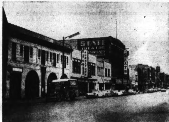
Section of South Saginaw to be rebuilt under the Urban Renewal Program.
