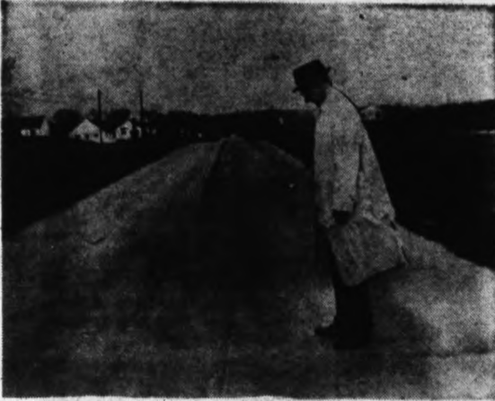
City Engineer James B. Carlisle inspects new concrete paving on Joslyn Avenue.
