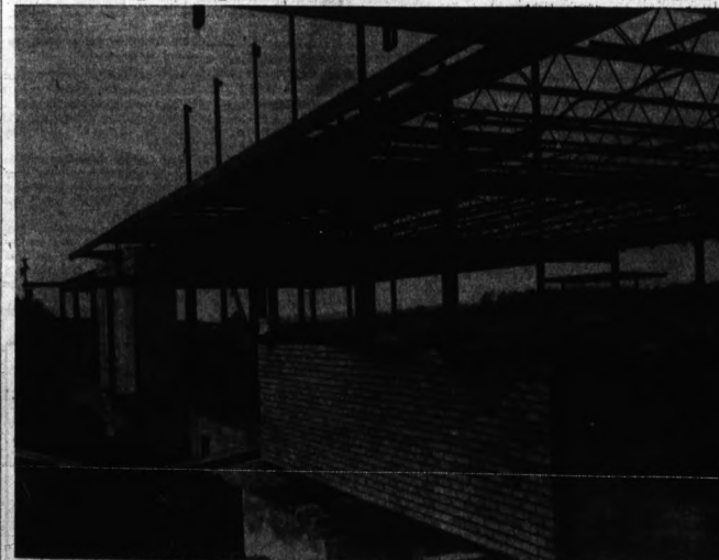
EYE SEPT. 1 COMPLETION DATE — Six weeks behind schedule because of bad weather and delays in steel delivery, the new terminal-tower building at Pontiac Municipal Airport begins to stand out against the sky. Homer D. Hoskins, airport manager, expects the time-lag will be made up this spring in time to finish construction on schedule Sept. 1. By next weekend, he said, the steel framework should reach as high as the fourth floor control tower. This view shows the eastern side of the growing, $346,000 building, with an indication (center) of its attractive brick exterior.
