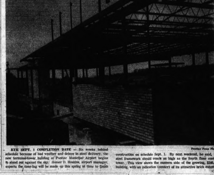
EYE SET. 1 COMPLETION DATE — Six weeks behind schedule because of bad weather and delays in steel delivery, the new terminal-tower building at Pontiac Municipal Airport begins to stand out against the sky. Homer D. Hoskins, airport manager, expects the time-lag will be made up this spring in time to finish construction on schedule Sept. 1. By next weekend, he said, the steel framework should reach as high as the fourth floor control tower. This view shows the eastern side of the growing, $346,000 building, with an indication (center) of its attractive brick exterior.
