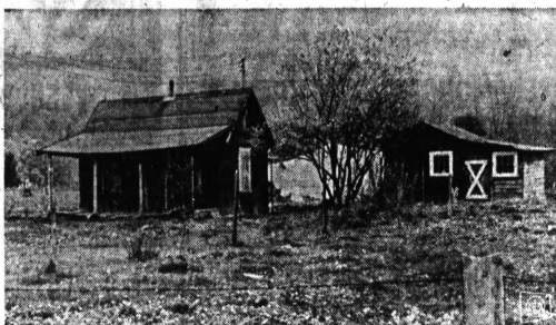
ONLY A SHANTY — A small tar paper house on the Seneca Indian reservation in Pennsylvania is typical of the tribe's homes.
