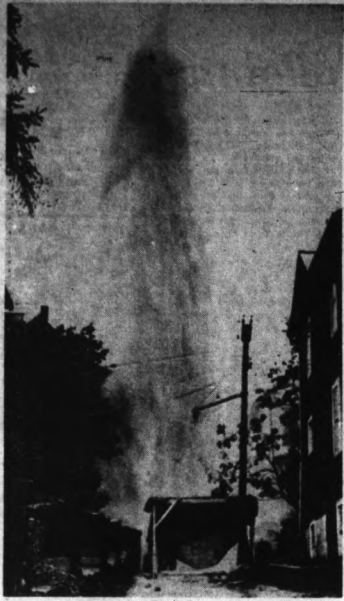
AP Photo THERE'S SIDE BLOW! — An impromptu geyser was created from the 66-inch main line from Quennahoning Dam to Bethlehem Steel's plant at Johnstown, Pa., when it broke Wednesday under a street. Sections of the plant were closed because of the lack of water. The gusher not only threw water more than 100 feet into the air but also carried with it stones and rocks, some of them bigger than a man's fist.
