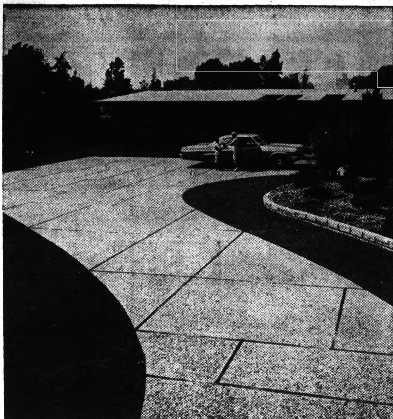
NO MORE MUD —A pebble concrete driveway blends naturally with lawn and shrubs. It has the hard durable surface of conven-
